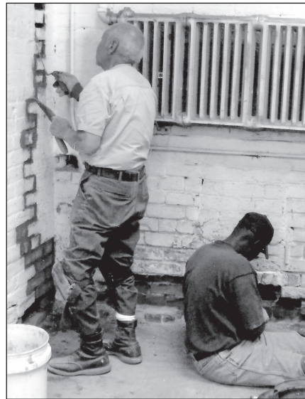
Don Calvert repairs the crumbling brick.
