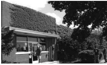
Corner Brewery, former Motor Wheel Office Building
